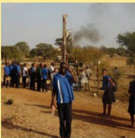
Drilling for a solar water pump in the Guénon school garden
