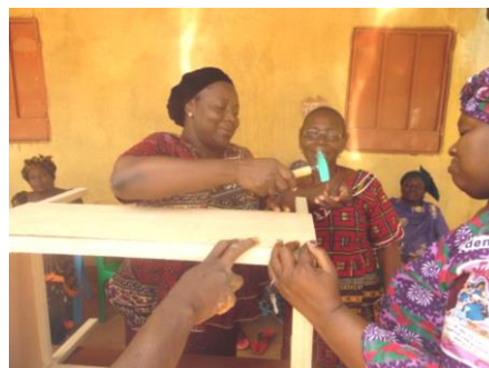
Great joint efforts: workshops for building your own solar oven
