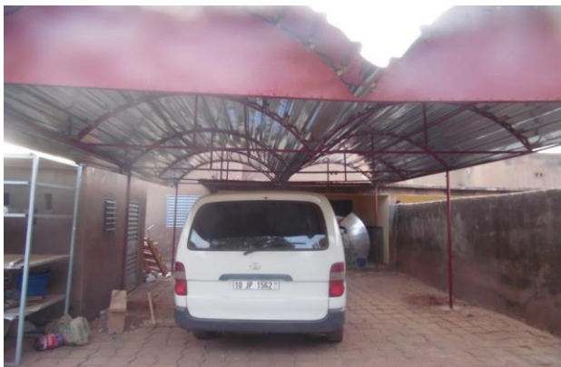
A new roof for better working conditions
