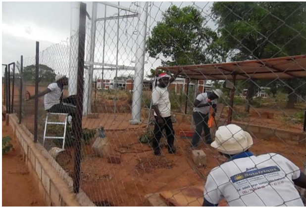
Repair work on a solar pump
