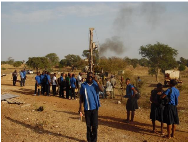
Students at the drilling site
