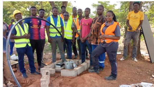
Installation der Pumpe in Bana2
