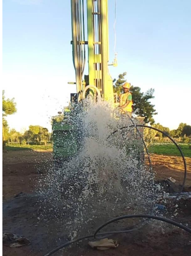
The result of a successful drilling
