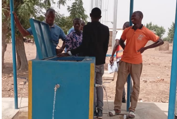
A new public water fountain, built by Solafrique
