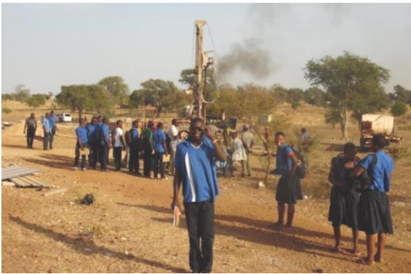
Drilling in Guénon
