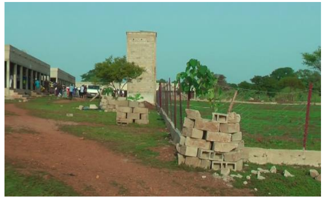
Water tower in Guénon
